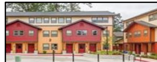
The Oaks at 14 th Permanent Supportive Housing
